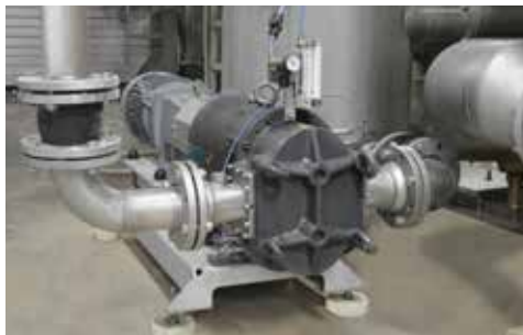
ONIXline pump for conveying Starch Slurry
