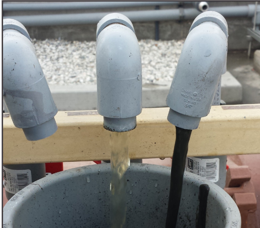
Low solids filtrate (left) is removed from digestate (right) while concentrated cake is returned to the digester.
