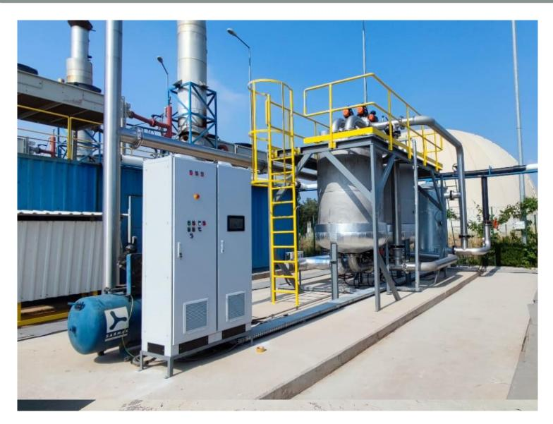
Landfill Gas Treatment System SGS-1400 is supplying clean gas for four of 1200 kW MWM type landfill gas engine for landfill gas to electricity power plant in Osmaniye. It has capacity of 1.400 Nm³/h gas flowrate. It started working in June 2022 and it is up and running now successfully.
