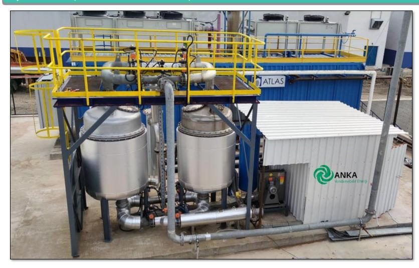
Landfill Gas Treatment System SGS-1400 is supplying clean gas for two of 1200 kW MWM type landfill gas engine for landfill gas to electricity power plant in Edirne. It has capacity of 1.400 Nm³/h gas flowrate. It started working in November 2020 and it is up and running now successfully.
