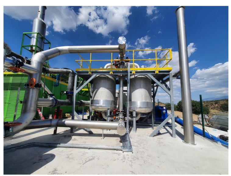
Landfill Gas Treatment System SGS-2500 is supplying clean gas for four of 1415 kW Jenbacher INNIO type landfill gas engine for landfill gas to electricity power plant in Manisa. It has capacity of 2.500 Nm³/h gas flowrate. It started working in June 2022 and it is up and running now successfully.
