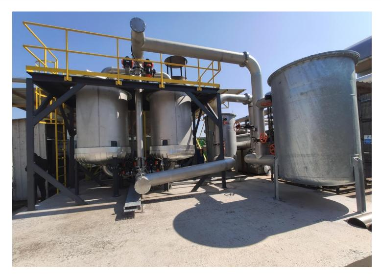
Landfill Gas Treatment System SGS-2500 is supplying clean gas for four of 1457 kW CAT type landfill gas engine for landfill gas to electricity power plant in Sakarya. It has capacity of 2.500 Nm³/h gas flowrate. It started working in March 2022 and it is up and running now successfully.
