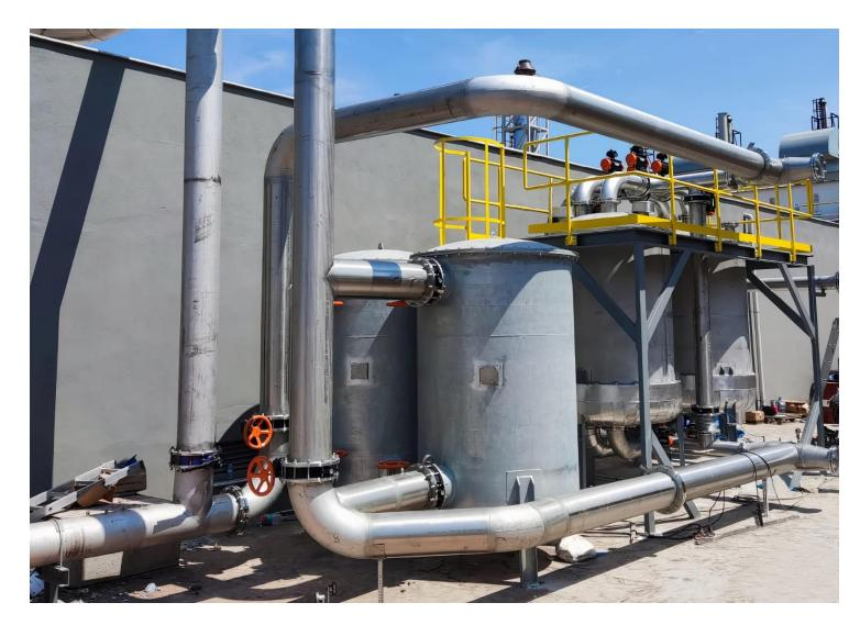
Biogas Gas Treatment System SGS-2500 is supplying clean gas for four of 1457 kW CAT type biogas gas engine for landfill gas to electricity power plant in Sakarya. It has capacity of 2.500 Nm³/h gas flowrate. It started working in July 2022 and it is up and running now successfully.
