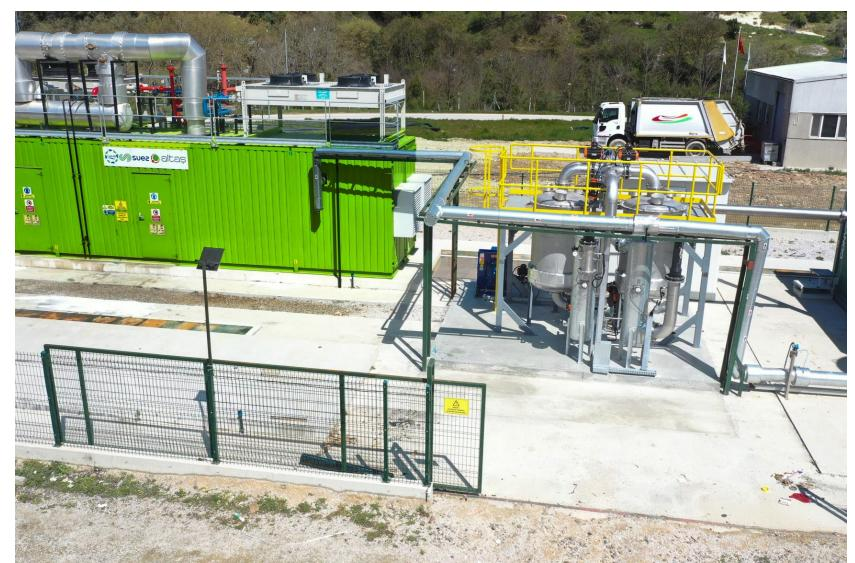
Landfill Gas Treatment System SGS-1400 is supplying clean gas for two of 1200 kW MWM type landfill gas engine for landfill gas to electricity power plant in Çanakkale. It has capacity of 1.400 Nm³/h gas flowrate. It started working in April 2022 and it is up and running now successfully.
