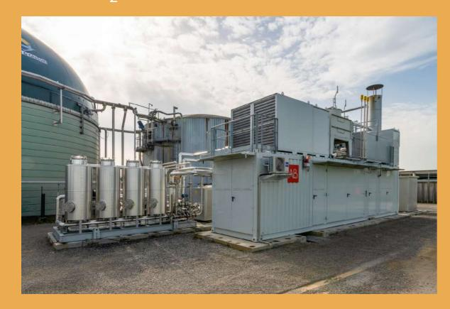
The DISCO<sub>2</sub>VERY CO<sub>2</sub> liquefaction system makes it possible to purify and liquefy the carbon dioxide-rich gas coming from the BIOCH4NGE<sup>®</sup> biogas upgrading system, in order to obtain liquid CO<sub>2</sub> suitable for food and industrial use.
