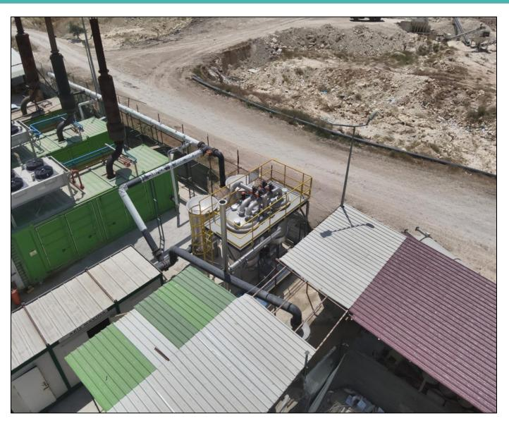
Landfill Gas Treatment System SGS-2500 is supplying clean gas for the 3.6 MW landfill gasto-electricity power plant in Silifke.
