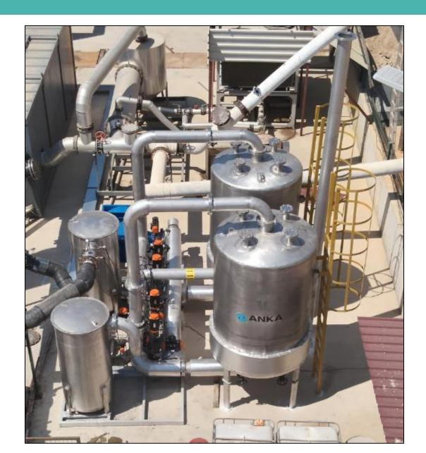
Landfill Gas Treatment System SGS-2750 is supplying clean gas for the Aydın landfill gas-to-energy plant operating with four 1.2 MW G56HM engines.
