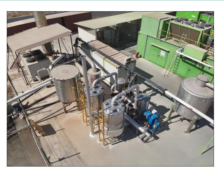
Landfill Gas Treatment System SGS-2000 is supplying clean gas for the Kuşadası Integrated Solid Waste Facility's power generation operations.
