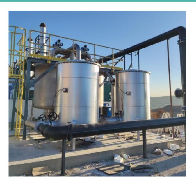
Landfill Gas Treatment System SGS-2500 is supplying clean gas for 4 of 1415 kW Innio Jenbacher type landfill gas engine for landfill gas to electricity power plant in Kayseri. It has capacity of 2.500 Nm3/h gas flowrate. It started working in January 2023 and it is up and running now successfully.
