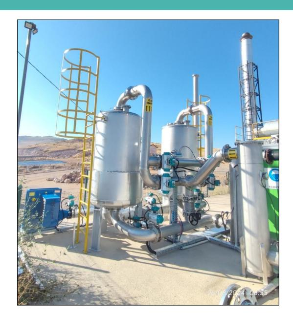
Biogas Treatment System SGS-900 is supplying clean gas for the 3.6 MW biogas-to-electricity facility in Nevşehir, which processes approximately 250 tons of municipal solid waste per day.
