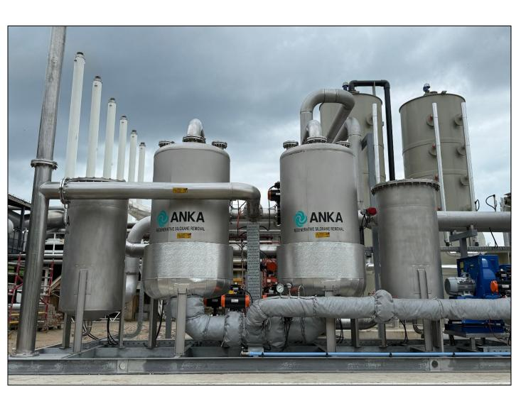
VOC Removal System SGS-1500 is supplying clean gas for the Riga landfill gas utilization facility in Latvia.
