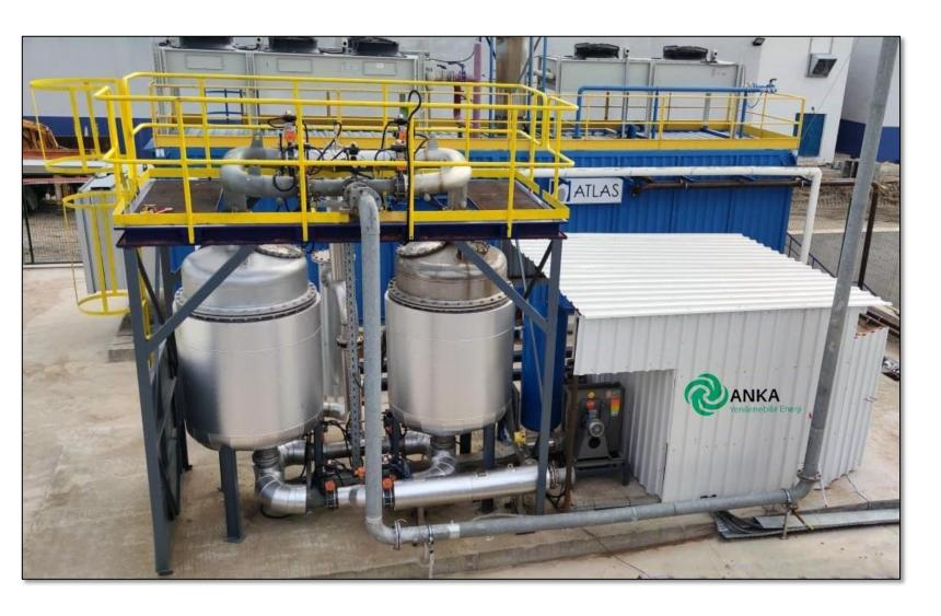
Landfill Gas Treatment System SGS-1400 is supplying clean gas for 2 of 1200 kW MWM type landfill gas engine for landfill gas to electricity power plant in Edirne. It has capacity of 1.400 Nm3/h gas flowrate. It started working in November 2020 and it is up and running now successfully.
