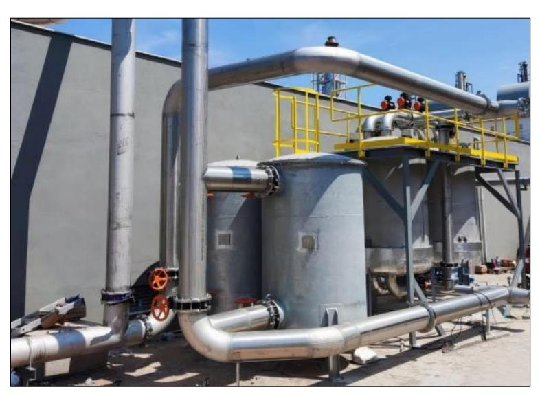
Landfill Gas Treatment System SGS-2500 is supplying clean gas for 4 of 1457 kW CAT type biogas engines for biogas to electricity power plant in Sakarya. It has capacity of 2.500 Nm3/h gas flowrate. It started working in August 2022 and it is up and running now successfully.
