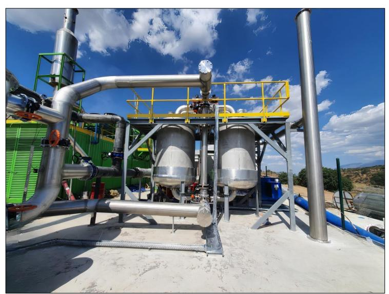
Landfill Gas Treatment System SGS-2500 is supplying clean gas for 4 of 1415 kW Jenbacher INNIO type landfill gas engine for landfill gas to electricity power plant in Manisa. It has capacity of 2.500 Nm3/h gas flowrate. It started working in June 2022 and it is up and running now successfully.
