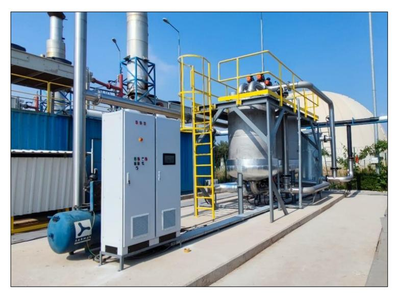
Landfill Gas Treatment System SGS-1400 is supplying clean gas for two of 1200 kW MWM type landfill gas engine for landfill gas to electricity power plant in Osmaniye. It has capacity of 1.400 Nm3/h gas flowrate. It started working in June 2022 and it is up and running now successfully.
