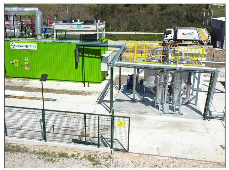
Landfill Gas Treatment System SGS-1400 is supplying clean gas for 2 of 1200 kW MWM type landfill gas engine for landfill gas to electricity power plant in Çanakkale. It has capacity of 1.400 Nm3/h gas flowrate. It started working in July 2022 and it is up and running now successfully.
