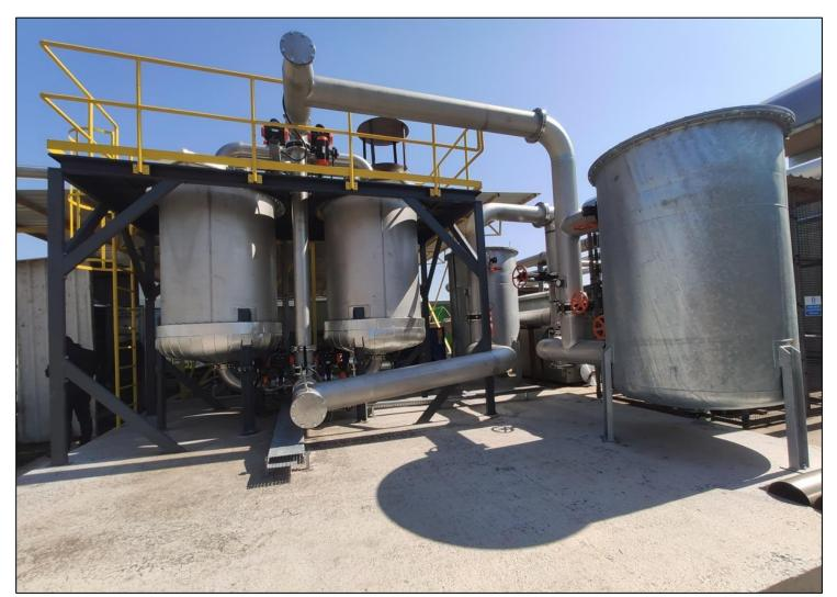
Landfill Gas Treatment System SGS-2500 is supplying clean gas for four of 1457 kW CAT type landfill gas engine for landfill gas to electricity power plant in Sakarya. It has capacity of 2.500 Nm3/h gas flowrate. It started working in March 2022 and it is up and running now successfully.
